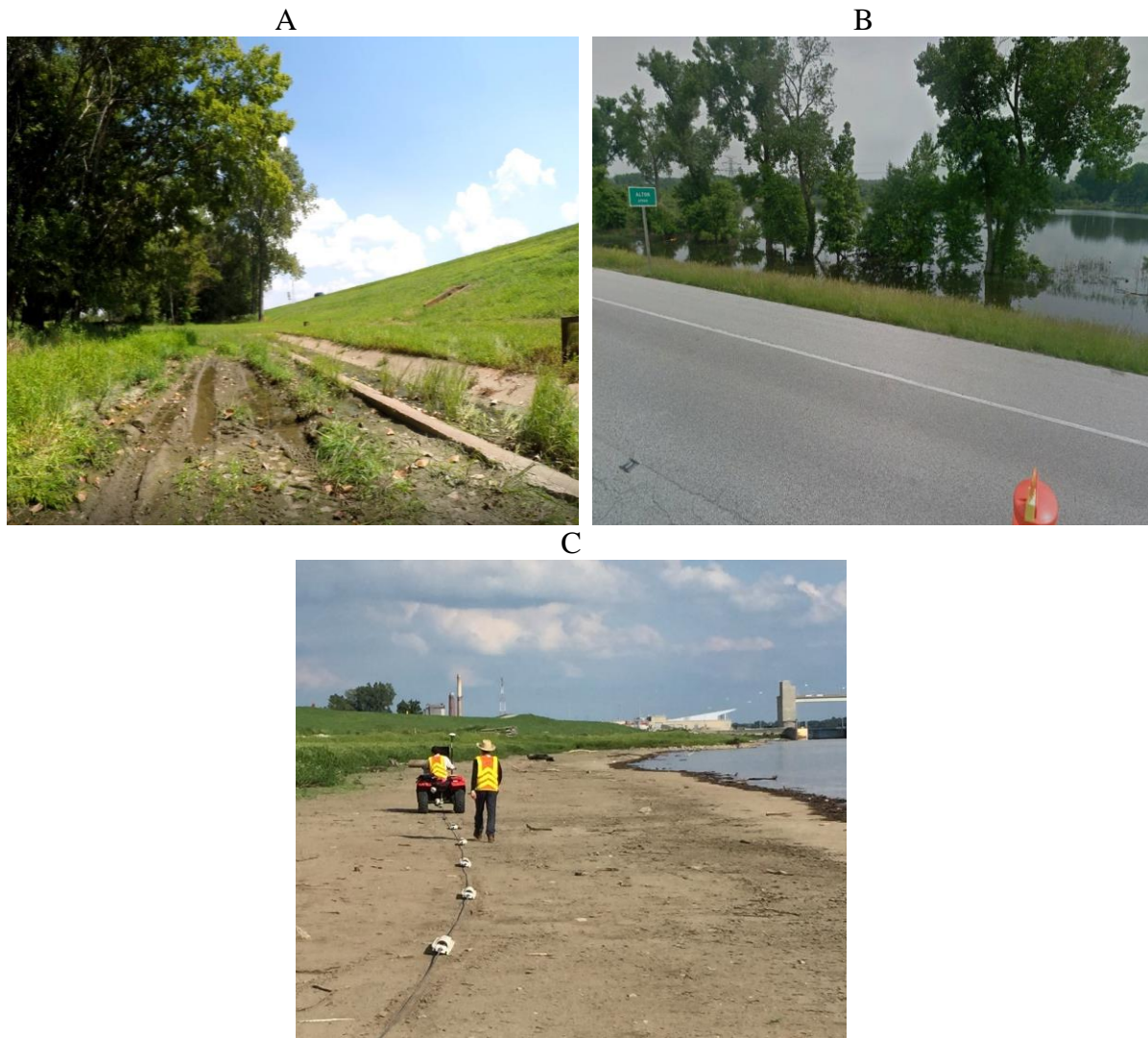
Figure 3-12. A) Visible surface water at landside of Mel Price Levee at sta. 123+00, B) View from top of road showing the pond along the landside of the Mel Price Levee at sta 95+00, and C) OhmMapper towed along riverside of Mel Price Levee at sta 82+00.
